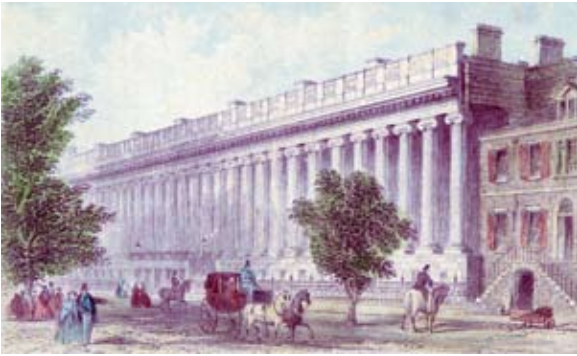
East front of the Main Treasury circa 1865. The 336-foot long colonnade, originally sandstone, was rebuilt with granite in 1908. On the right stands the old State Department building, which was razed in 1866 to make room for the north wing of Main Treasury. (Treasury Collection)
